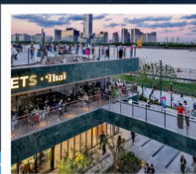
GATE M WEST BUND
