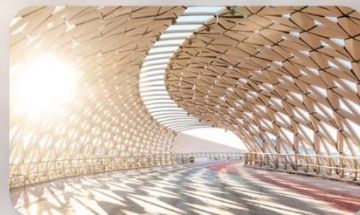
Ayrau Bridge Astana
