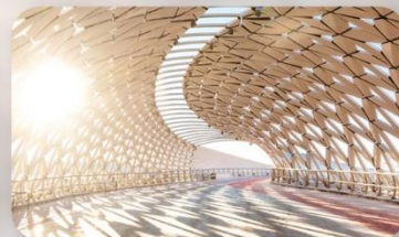
Ayrau Bridge Astana
