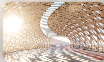
Atyrau Bridge Astana
