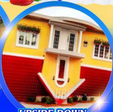
UPSIDE DOWN HOUSE
