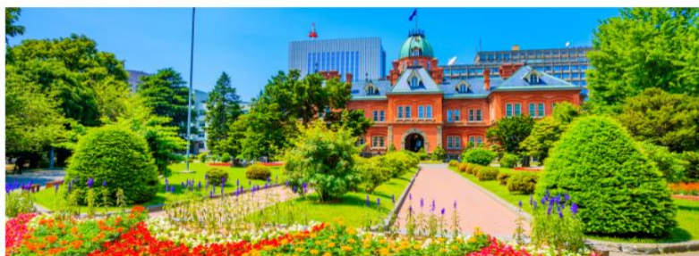
FORMER HOKKAIDO GOVERNMENT OFFICE BUILDING
