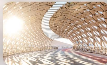
Ayrau Bridge Astana
